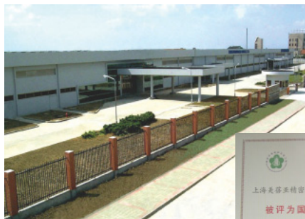
Xicen Factory, Minebea Electronics & Hi-Tech Components (Shanghai)
